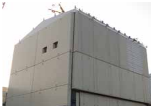
Unit 1 reactor building cover installation
