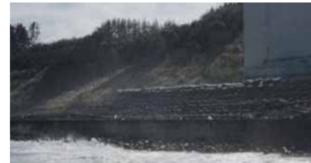
Installation of temporary tide barrier
