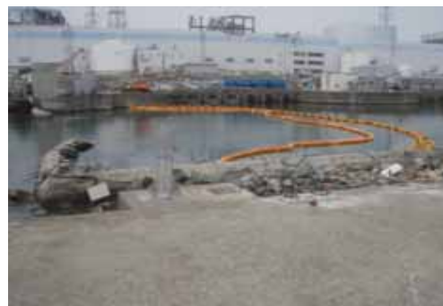
Silt fence installation
