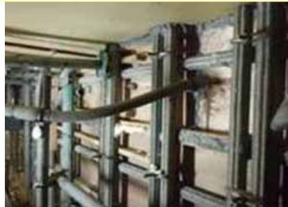
Injecting grout (Jul. 30)
