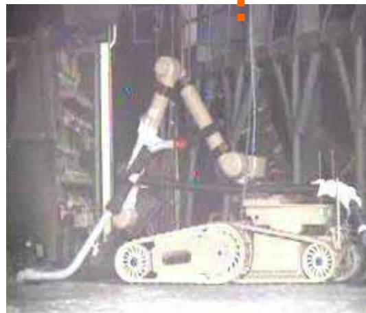
Cleaning in Reactor Building of Unit 3 (July 1)
