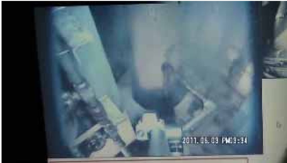
Steam release from the penetration on 1 st floor (photo as at Jun. 3)
