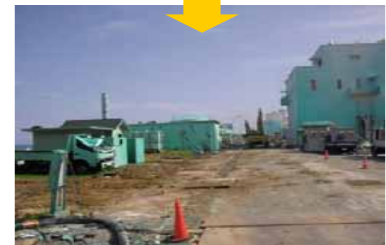
Removal of rubble
